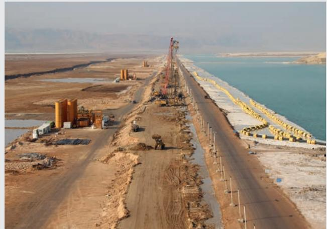
The subsoil presented a special challenge: The hard crystalline salt layers required the use of two Bauer cutter units, in combination with one grab unit. Also, the tremendously critical effect of the high salt content on the support fluid had to be addressed by developing innovative custom-made compositions.
