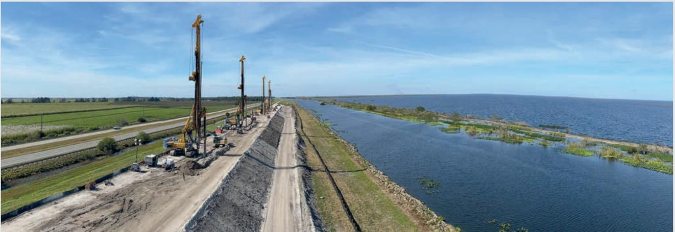
***Bauer is proud to have been contracted to execute many cut-off wall projects as part of the Herbert Hoover Dike Rehabilitation in FL, USA. Working both as a General Contractor for the US Army Corps of Engineers or as a Subcontractor. Nearly 28 miles of CSM (over 5 million square feet!) have been installed, starting in 2008 with the Reach 1 task orders, continuing through 2019 with various new culverts and continues into 2022 with the multiple award task orders.***
