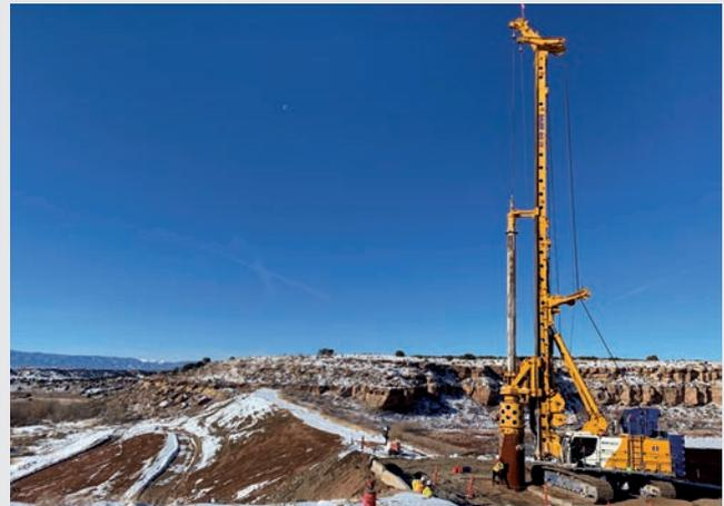
Casing installation with the rotary drive of the drill rig (pushing and rotation).
