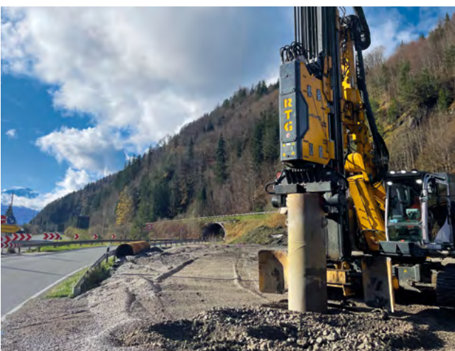
New construction B2, Eschenlohe, Germany For the new B2 bypass, a total of 6,200 m of vibro textile columns were constructed.
