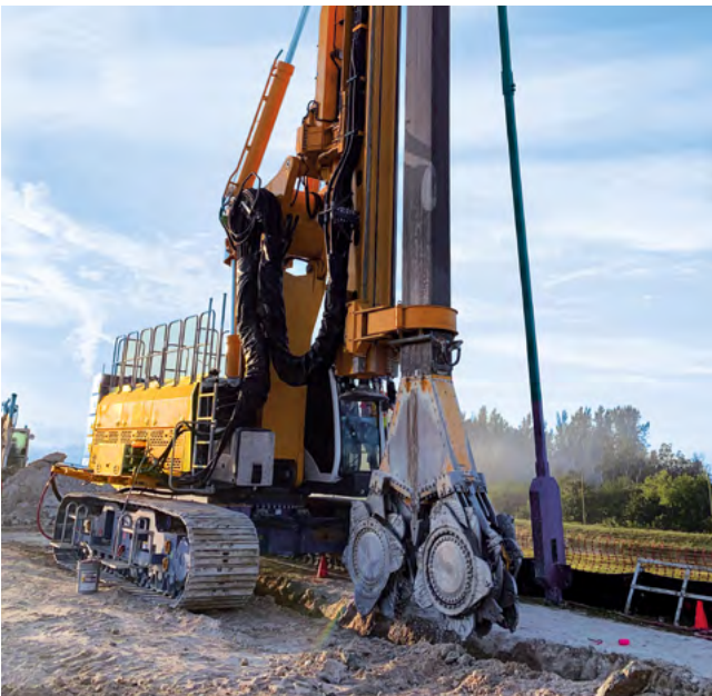
Herbert Hoover Dike, Florida, USA To improve dam security, a 28.3 km cut-off wall was installed with a depth of up to 20 m.
