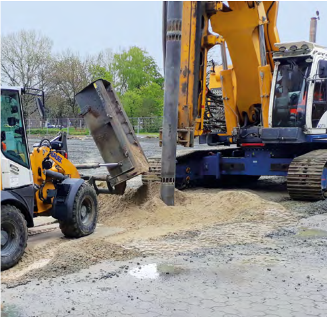
Center for Deep-Sea Research (Zentrum für Tiefseeforschung – ZFT), Bremen, Germany For the new ZFT building in Bremen, Bauer executed 5,500 m of vibro compaction work.
