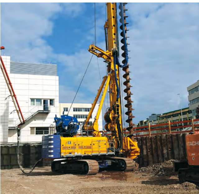
New building of central laboratory, Herzogenaurach, Germany Drilling of foundation piles with a diameter of 1,000 mm and depth of 18 m using the CFA method.
