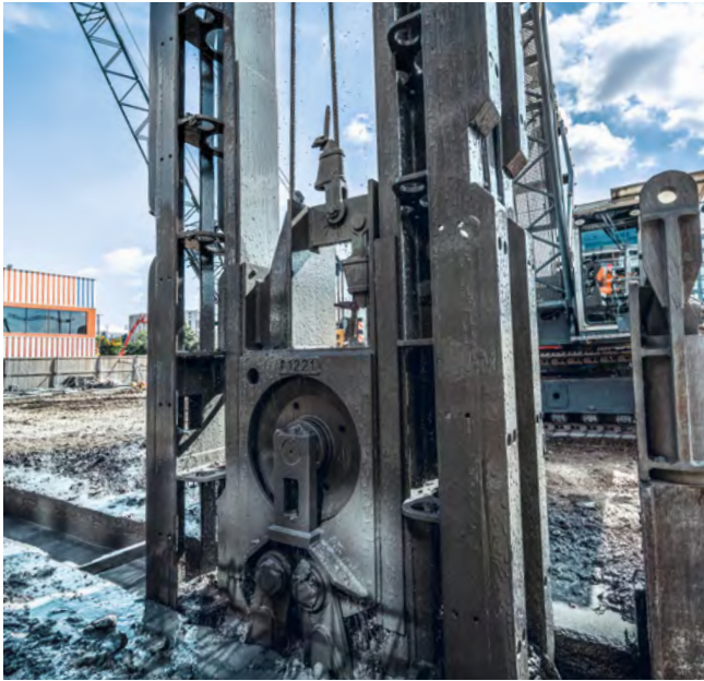
South entrance to exhibition grounds, Frankfurt am Main, Germany Execution of a 2-phase diaphragm wall using an MC 64 duty-cycle crane with grab.
