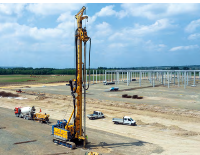
New construction of logistics halls, Maglód, Hungary Construction of foundation piles with a diameter of 360 mm using FDP method.
