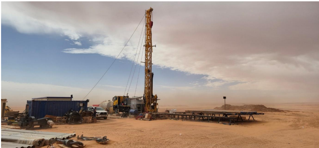
(2) During the first phase, the RB 50 rigs will drill 710 groundwater wells within two years under challenging climatic conditions.
