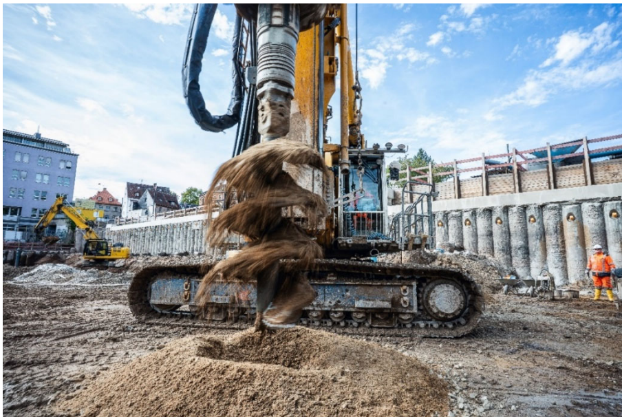
(3) Powerful: A BAUER BG 39 constructing piles for the foundation.
