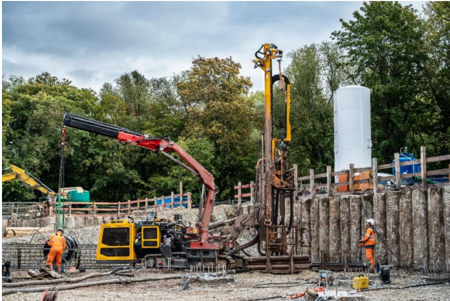
(2) A well-coordinated team: Geothermal work and specialist foundation engineering go hand in hand on this project.
