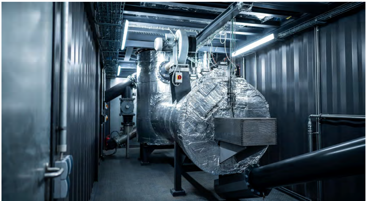
The pyrolysis plant from Carbo-FORCE carbonizes biomass.
