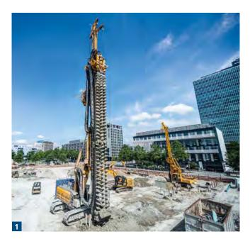
**1 Parkstadt Schwabing, Munich:**For a 9 m deep excavation pit, Bauer constructed a 6,000 m<sup>2</sup> single-anchored Mixed-in-Place cut-off wall.
