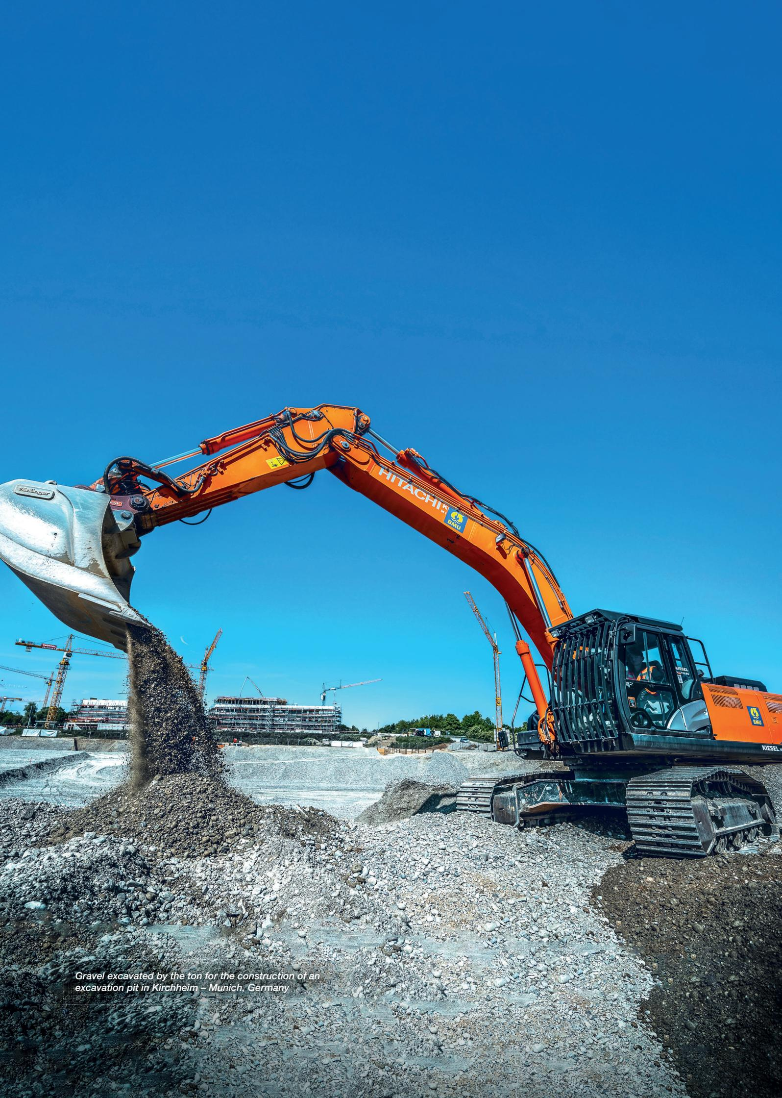
*Gravel excavated by the ton for the construction of an excavation pit in Kirchheim – Munich, Germany*
