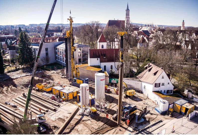
In **Schrobenhausen**, the home-town of Bauer, a new residential complex with two houses and a total of 2,400 m<sup>2</sup> living space will be created by 2021. To seal against ground water, the excavation pit was made impermeable before excavation with a retaining wall using a combination of sheet pile wall construction and the Mixed-in-Place method. **top**
