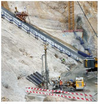
**Lebanon** The Jannah Dam northeast of Beirut serves as a reservoir for the region. To seal the dam and grout the rock in sections of the foundation that are subjected to high pressure, Bauer carried out approx. 25,650 m of injections. **top**
