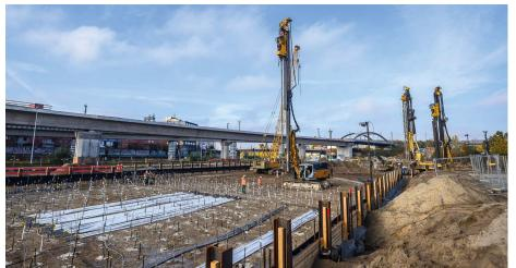
An environmentally sound and sustainable LWS silicate gel base was used for the horizontal seal of the excavation pit for the QH Track project in Berlin, comprising around 16,000 m<sup>2</sup>.
