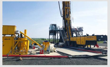
**Italy** For a project in the harbor of Trieste, I.CO.P. S.p.A. used a BG 24 H to manufacture a cut-off wall, using the SCM method. **bottom**
