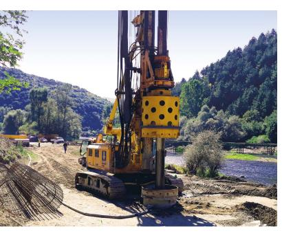
**Bulgaria** Good planning and organization was required for the execution of large-diameter bored piles for the Zheleznitsa Tunnel, which will be the longest tunnel in Bulgaria when it is completed. Piles with a diameter of 1,500 mm and 1,800 mm were installed up to a depth of 25 m. **top**
