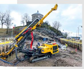
**Sweden** To secure a sheet pile wall with self-drilling anchors, our customer NCC in Gothenborg relied on a KLEMM KR 806-5G. **top**
