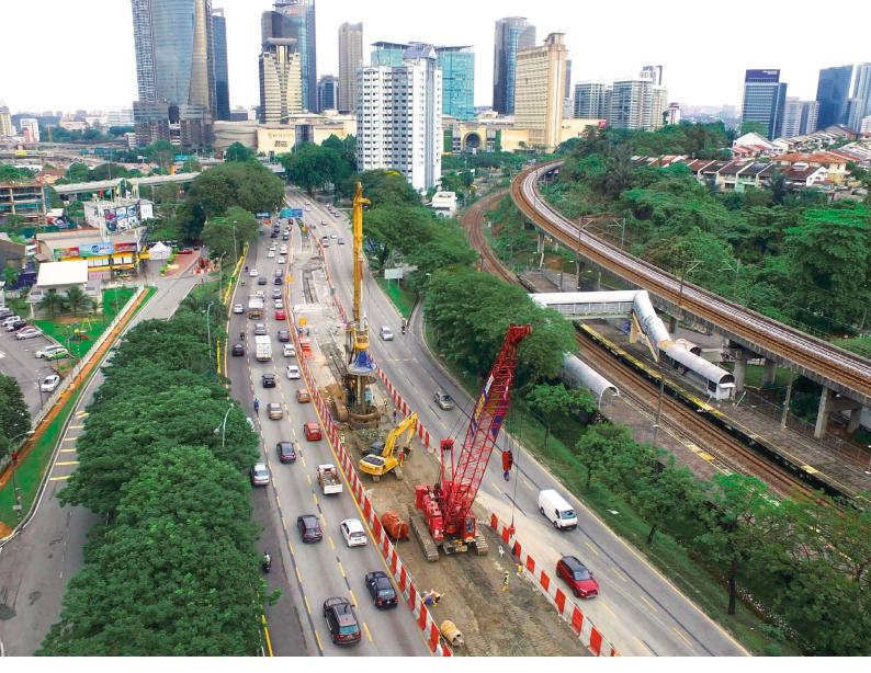
**Malaysia** For the new Setiawangsa-Pantai Expressway under construction to improve the traffic situation in Kuala Lumpur, 56 foundation piles were constructed using a BG 40 and BG 45. **top**
