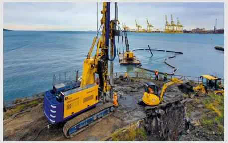
**Monaco** The construction of piles in the harbor of Monaco was successfully concluded by the company Fondamenta S.r.l. using a BG 55 and a BG 45. **bottom**
