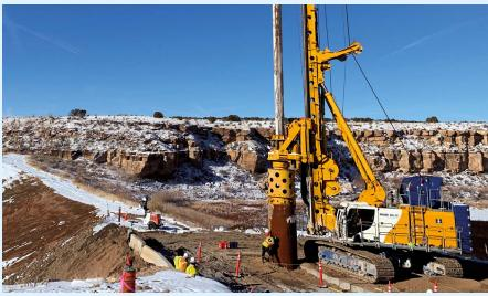
**USA** The Teller Dam is located within the U.S. army base Fort Carson near Colorado Springs. Bauer was contracted to seal the dam and will construct approx. 1,160 m<sup>2</sup> of secant pile wall as well as approx. 1,760 m<sup>2</sup> of grout curtains for this purpose. **top**
