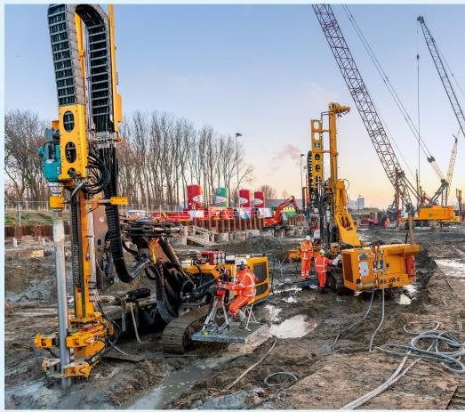
**Netherlands** For a new motorway link in Rotterdam, around 10,000 t of material were installed in the second-largest city in the Netherlands. A total of 4,500 GEWI<sup>®</sup> thread bar piles, that is, micro piles with threads, were required for the "Blankenburg connection" and executed by a total of eleven teams using eleven KLEMM KR 806 rigs. **top**
