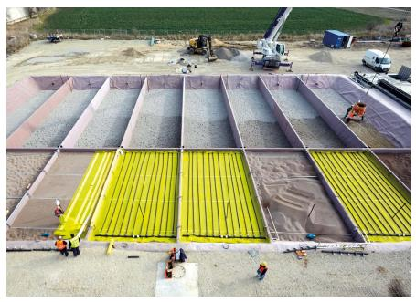
A large-scale plant has been operating since 2014 based on the EcoVert<sup>®</sup> method to clean approx. 22 m<sup>3</sup> per hour of highly contaminated ground water from a former refinery location.
