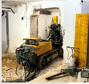
**Italy** Our customer Brenelli Costruzioni S.r.I. installed micropiles in the ground of a basement, using a KLEMM KR 702-2 and a KR 802-3S. **top**
