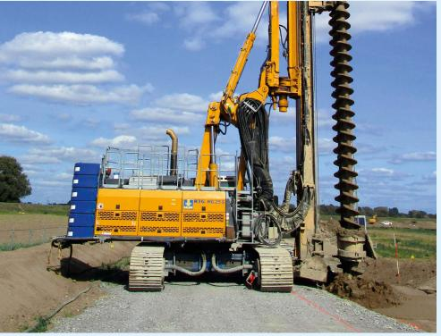
To permanently protect the banks of the Rhein against flood, Bauer Spezialtiefbau constructed a new cut-off wall for dike relocation near the district of **Mündelheim** in Duisburg. Over a length of 1.6 km, a total of approx. 28,000 m<sup>2</sup> of cut-off wall was constructed up to a depth of 20 m using the Mixed-in-Place method. **left**
