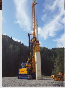
**Norway** The customer Keller Grundbau executed a bridge construction site with a BG 36 using the Kelly drilling method. **top**
