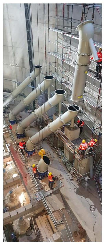
The installation of pipe work on the pressure side in the Oberhausen pumping station requires the utmost precision (left), as does pipeline installation with heat exchangers (bottom).
