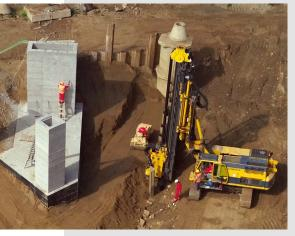
**Greece** For the pile foundation of an industrial complex, our customer Triantafillakis Foundation Works used a BG 24 H as well as a BG 20 H. **bottom**
