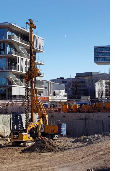
The new construction of a residential and commercial building in **Munich** will establish 164 apartments, a day-care center, and an underground garage. Bauer Spezialtiefbau was commissioned to construct 6,900 m<sup>2</sup> of static MIP wall as well as 650 running meters of anchors with five to six strands. **bottom**
