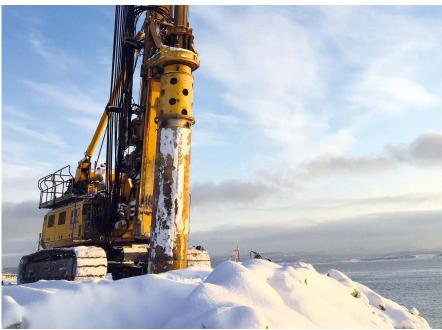
**Russia** For a new ocean engineering center in the Russian city of Murmansk, Bauer created a total of 2,540 lin.m. of piles with a length of up to 32 m. Construction was completed after 50 days of work. **top**
