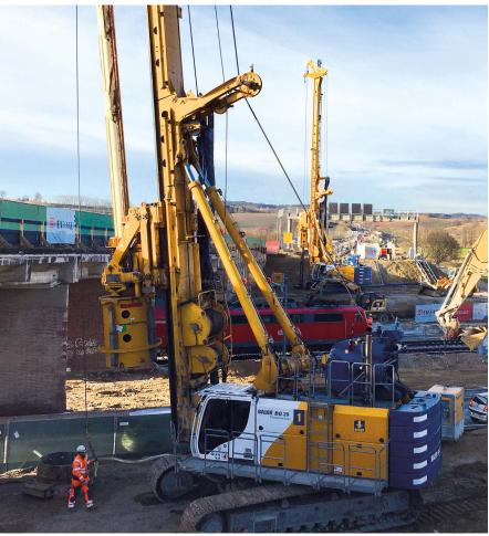
Using a BG 30, an excavation pit was created in **Mainz** for a residential building and hotel. First, 370 foundation piles were installed using the CFA method with drilling depths of up to 20 m, followed by retrofitting for the Kelly drilling method. **right**
