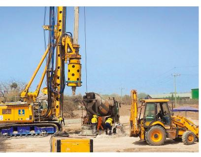
**Burkina Faso** A secant pile wall created using the Kelly drilling method up to a depth of 23 m forms the foundation for a new mine ventilation shaft. **top**
