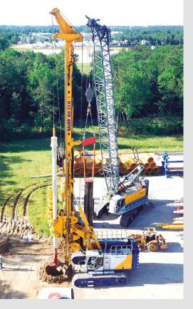
**China** On the Xin River, Jiangxi Bingxin constructed a cut-off wall with a BG 38, using the CSM method and an eccentric screw pump EP 14-400 from MAT. **bottom**
