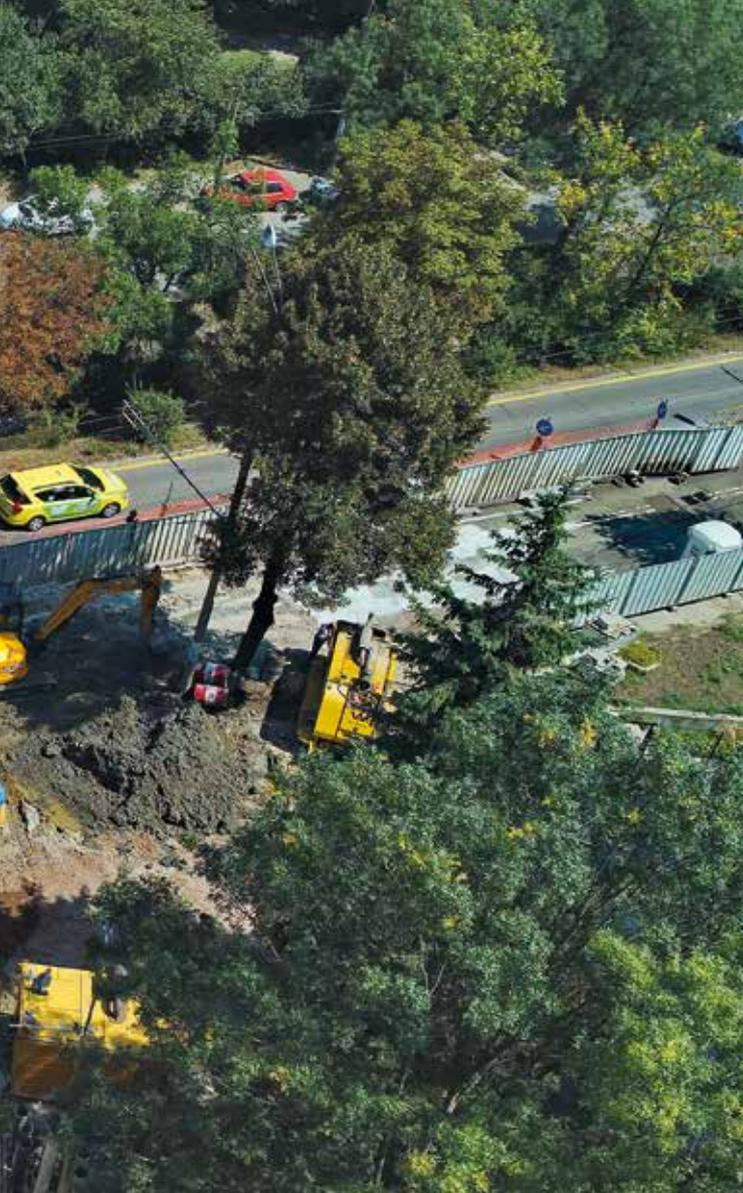
**Hungary** For a new sports center in the heart of Budapest, roughly 2,000 m<sup>2</sup> of diaphragm wall was built down to a depth of 20 m in tight space conditions. The earth works involved excavating around 11,000 m<sup>3</sup> of soil down to a depth of 18 m below ground level – not an average excavation depth for Hungary. **Bottom**
