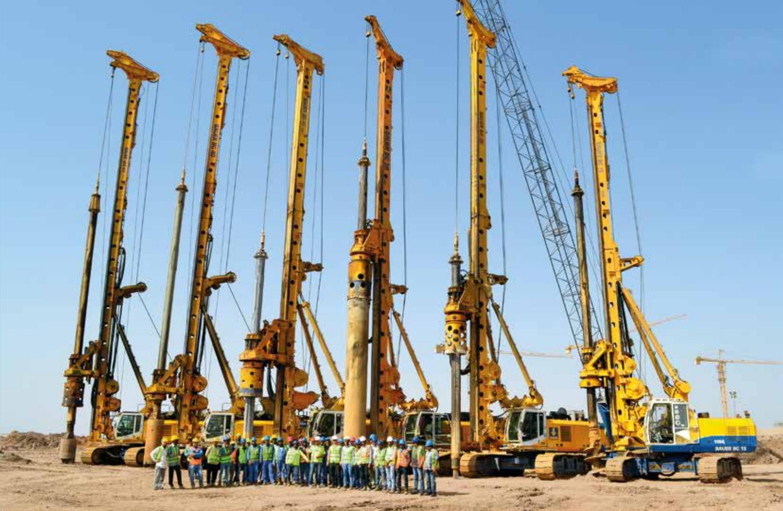
**Saudi Arabia** Seven drilling rigs, comprising of models BG 15, BG 28 and BG 40, are being used for the foundation works for a medical center in Jeddah. Over 200 employees are involved in building the foundation and shoring piles. **Top**
