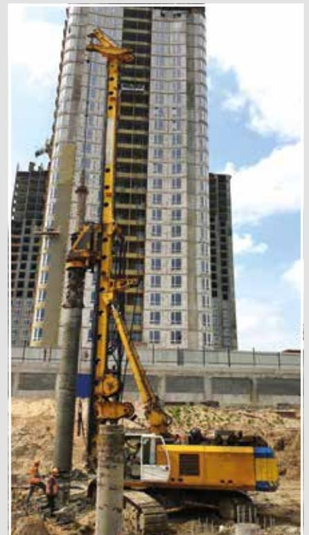
**Austria** Geops Bohrgesellschaft mbH used a KLEMM KR 805-3G for a dewatering well drilling with stand pipe for a tunnel. **Top**
