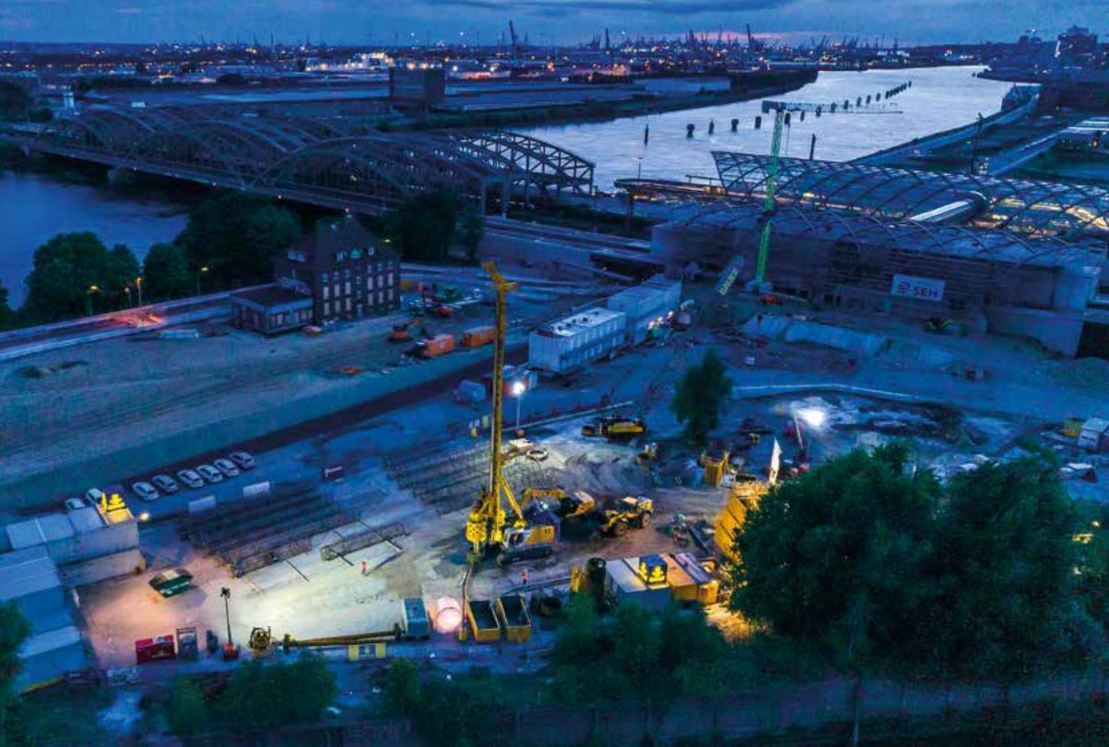
When drilling a test pile trial for the Elbtower **Hamburg** mega-project in the new HafenCity district, the Bauer team set a new record and installed the deepest pile in Germany, at 111.4 m. **Top**
