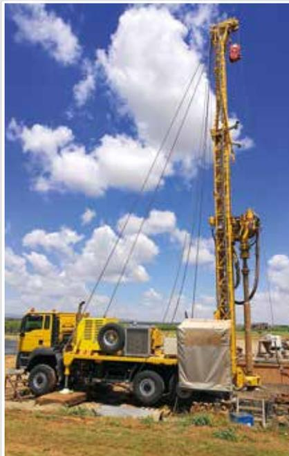
**Turkey** Our customer Sezerler Zemin Ins. San. Tic. Ltd. Sti. drilled multiple piles to protect a pipeline against landslides using a BG 28 H with Kelly equipment. **Bottom**
