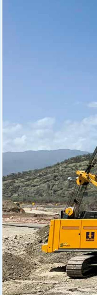
**Panama** To protect the Pedro Miguel locks on the Panama Canal against erosion, a BG 28 was used to build a secant pile wall consisting of 302 piles. **Right**
