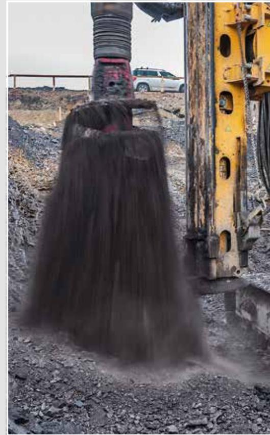
**Czech Republic** For the pile foundation of a high-rise office building in Prague, our customer Hinton a.s. used a BG 24 H with Kelly equipment. **Top**
