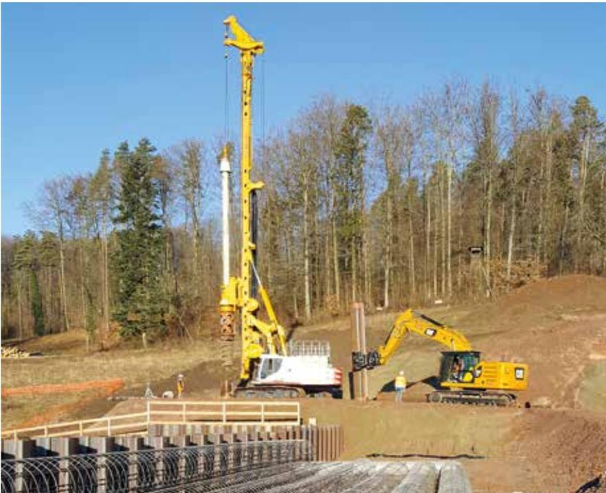
In **Schwörstadt**, as part of a deodorizing plant for a gas transmission network operator, Bauer constructed roughly 3,500 m<sup>2</sup> of tied-back sheet pile wall for site profiling and 700 running meters of pile foundations. The work was performed under strict safety precautions because some of the nearby high-pressure gas lines were still in operation. **Top**
