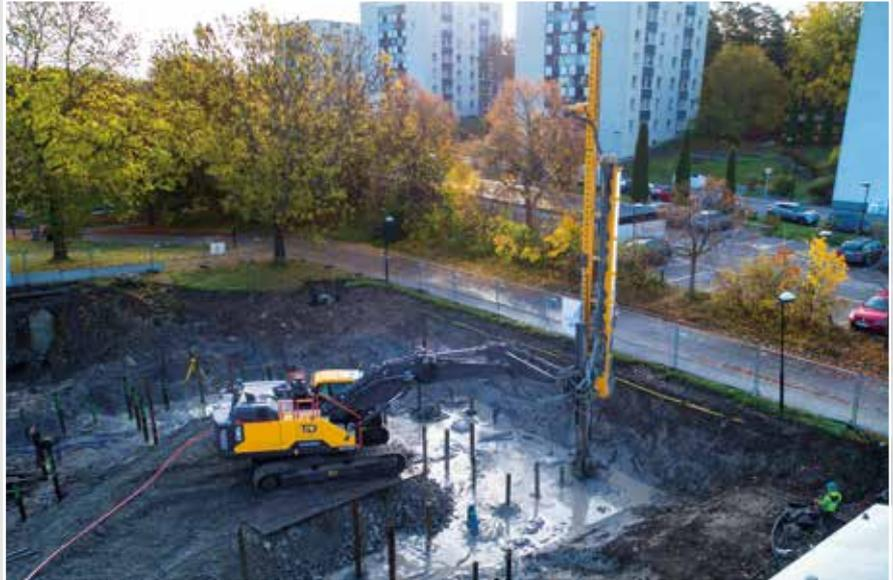
**Belgium** When restoring a church near Brussels, our customer CVR nv. opted for a Klemm KR 801-3FS for micro-pile drilling. **Bottom**
