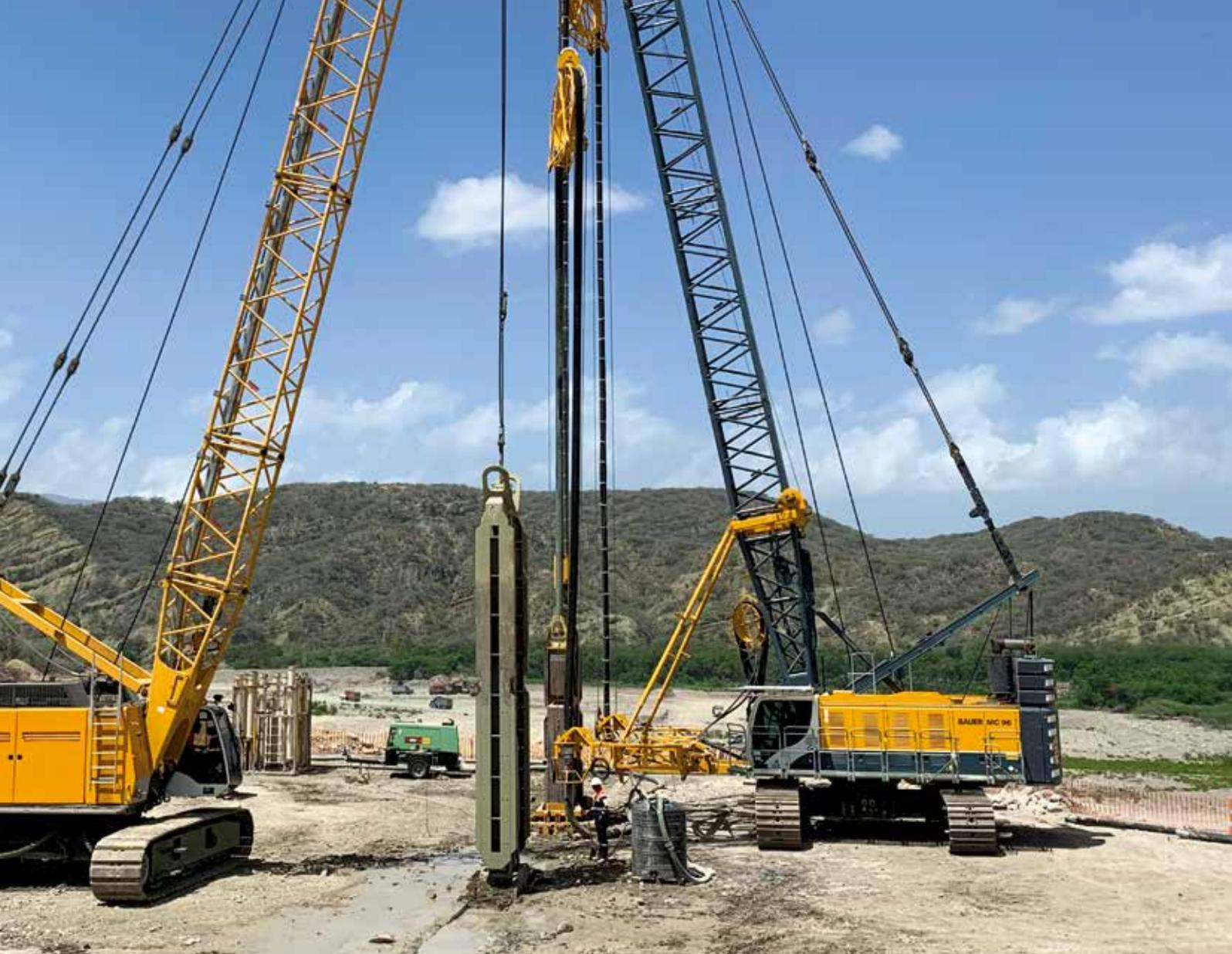
**Dominican Republic** To construct the new Monte Grande Dam on the Yaque del Sur River, roughly 30,000 m<sup>2</sup> of cut-off wall are being built down to a depth of 30 m. The works are being implemented with an MC 96 duty-cycle crane with a BC 40 cutter. **Top**
