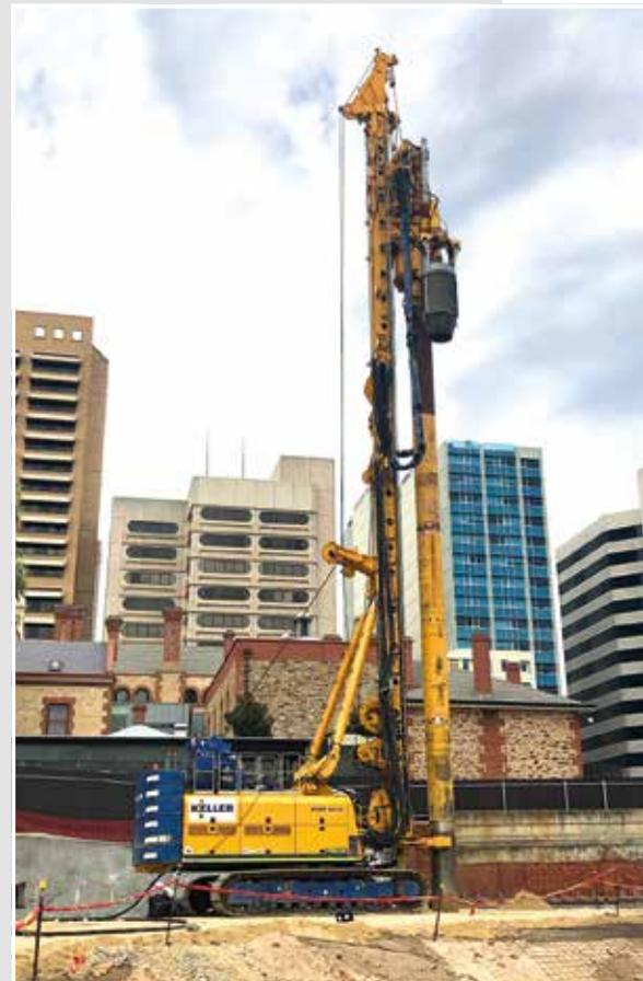
**Australia** In Adelaide, Keller Australia used a BG 30 equipped with a cased continuous flight auger to build a five-story car park. **Top**
