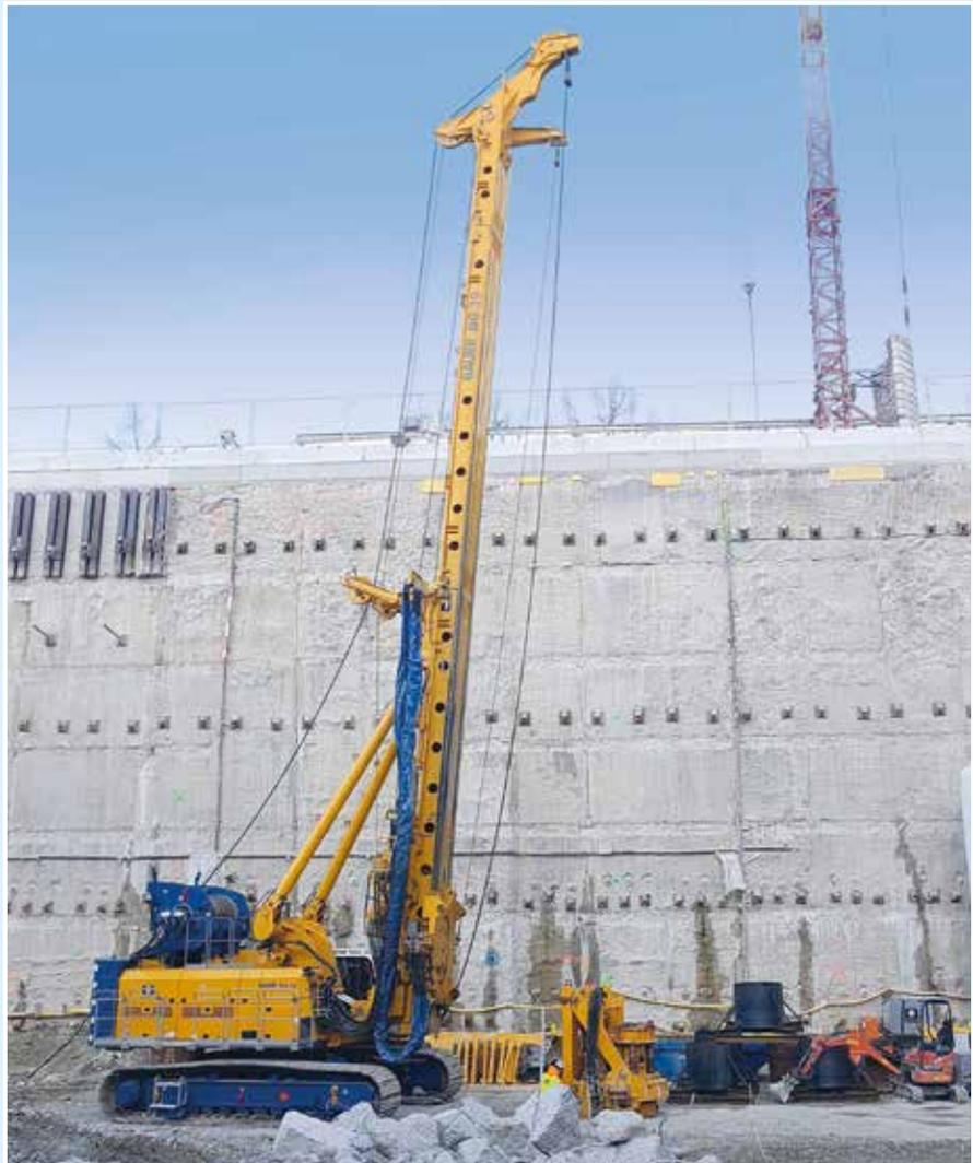
**Switzerland** For a new international research and development center for F. Hoffmann-La Roche AG in the city center of Basel, roughly 5,000 m of cased cast-in-situ piles were installed down to a depth of 35 m. **Top**
