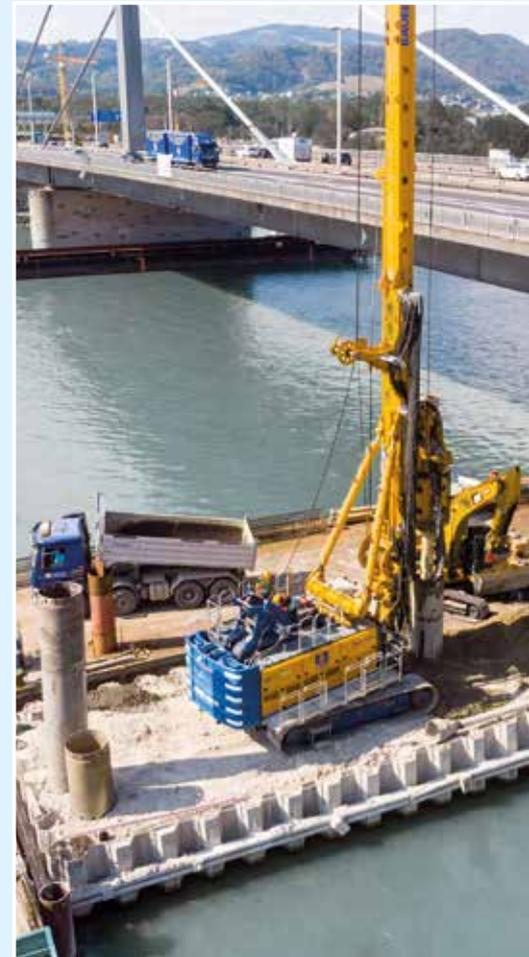
**Netherlands** To remediate the existing Amstelveen tram line in the south of Amsterdam, Bauer built approximately 1,200 GEWI® piles. The tram line was shut down temporarily for the works. **Top**
