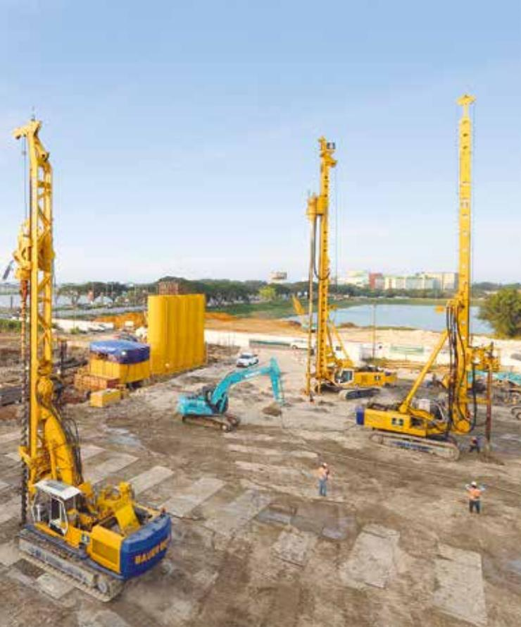
**Malaysia** No less than three records were broken during the piling works as part of the Lot L&M project in KLCC – Kuala Lumpur City Center. For the skyscrapers, Bauer drilled the deepest piles in Malaysia to date using the currently largest Bauer drilling rig BG 72 and the world's longest kelly bar at 150 m. **Bottom**
