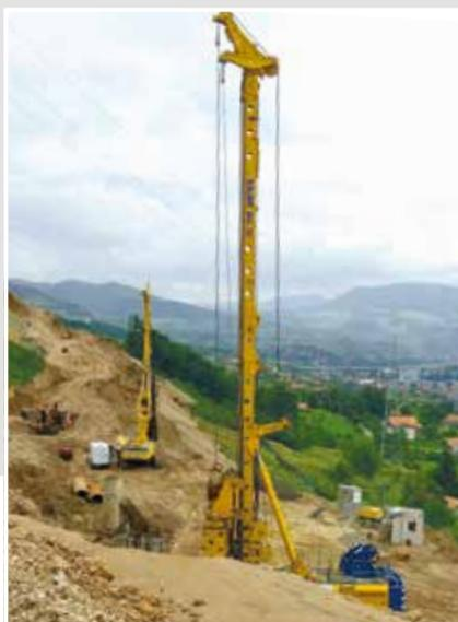
**Germany** Porr Equipment Services GmbH used a BG 45 V with Kelly equipment to build a secant pile wall for a hydroelectric power plant on the River Inn. **Top**
