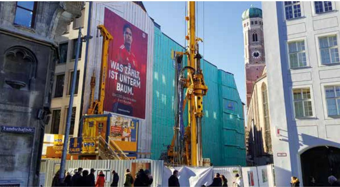
Using a BG 30 and a BG 15 H and applying the front-of-wall method, a retaining structure was built down to a depth of 18 m in the center of **Munich**, between the town hall and Frauenkirche church.
