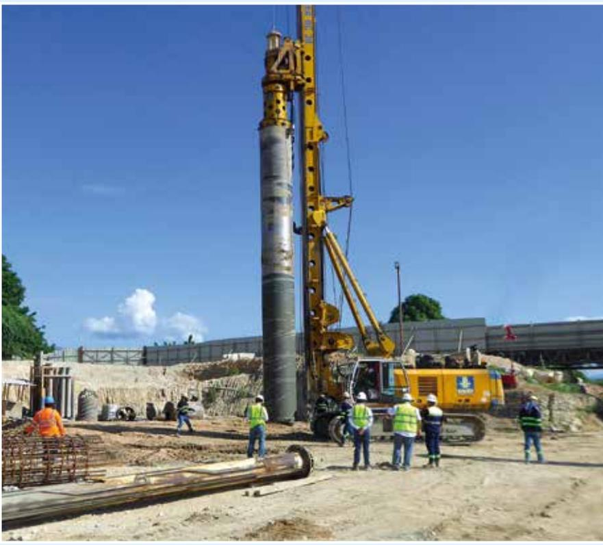
**Haiti** In Port-au-Prince, Bauer drilled a total of 97 piles for the foundations of two bridges across the Grey River. The BG 28 was brought in from the Dominican Republic for the works. **Left**
