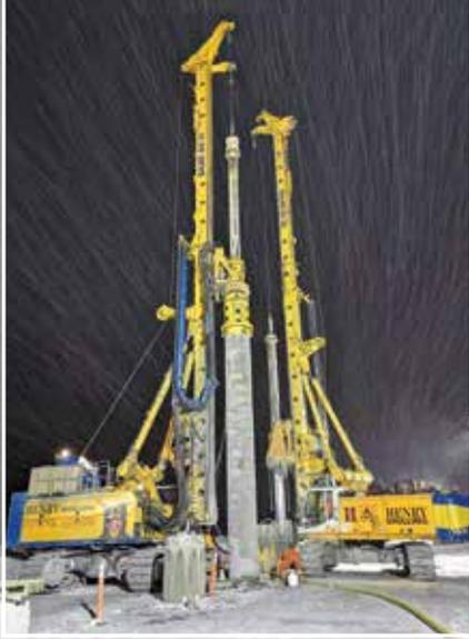
**Canada** Our customer Henry Drilling used two BG 30 V and a BG 28 V to build a secant pile wall in the Canadian tundra in Nunavut. **Top**
