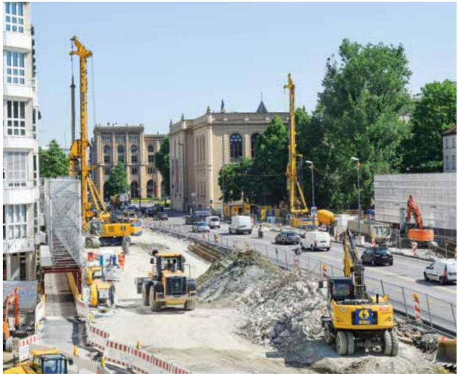
*Specialist foundation engineering and earth works for a multi-storey underground parking garage under the eastern Altstadt ring road in Munich.*
