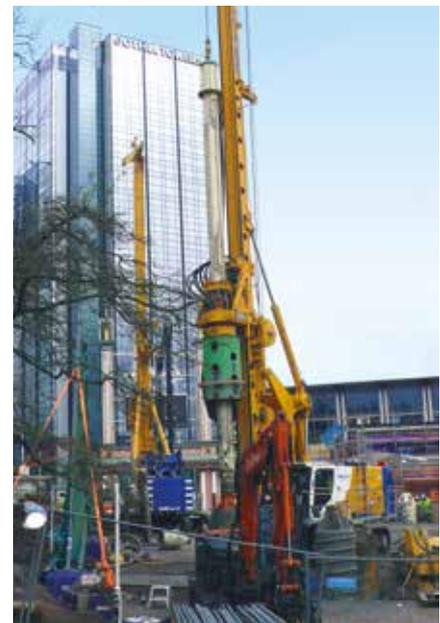
**Sweden** To secure a tunnel portal for the new subway in Gothenburg, Bauer built a pile wall consisting of roughly 60 piles down to a depth of 35 m to the left and right of the subway line. **Top**
