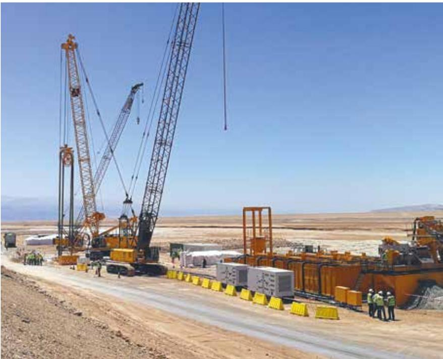
**Jordan** To seal earth basins used to create potash via condensation of salt water from the Dead Sea, around 112,000 m<sup>2</sup> of diaphragm wall is currently being built with embedded sheet pile walls. Additionally, 790,000 m<sup>3</sup> of soil must be moved in order to widen the dike. **Top**
