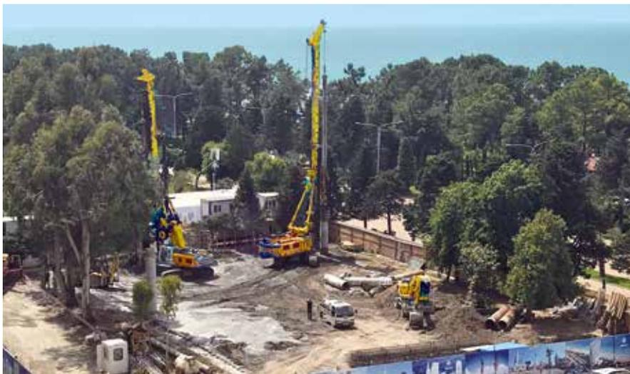
**Georgia** For a recreation center with a hotel on the exclusive Batumi Boulevard by the Black Sea, the deepest and largest pile ever drilled in Georgia was installed at a length of 62.3 m and a diameter of 1,500 mm. **Top**
