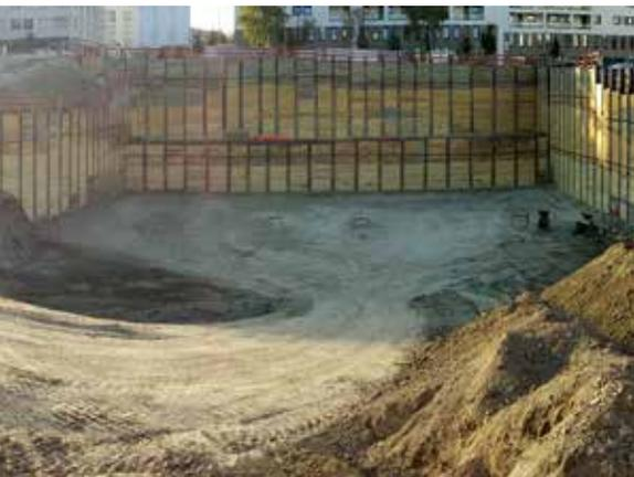
A new building project combining urban living and a green environment is being built in **Stuttgart**. In total, Bauer installed 3,300 m<sup>2</sup> of composite retaining wall with 127 soldier beams down to a depth of 18 m. **Top**
