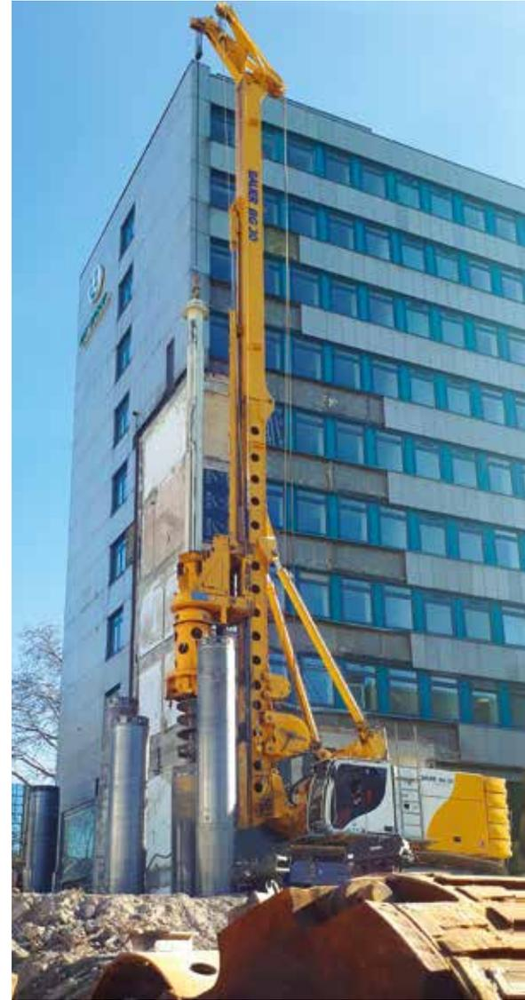
After decontamination and demolition of the existing structure, 1,550 m<sup>2</sup> of pile walls and 1,680 m<sup>2</sup> of contiguous pile walls with shotcrete gap filling were built for the Huyssen Quartier in **Essen**. The spatial restrictions in the city center were a particular challenge. **Top**
