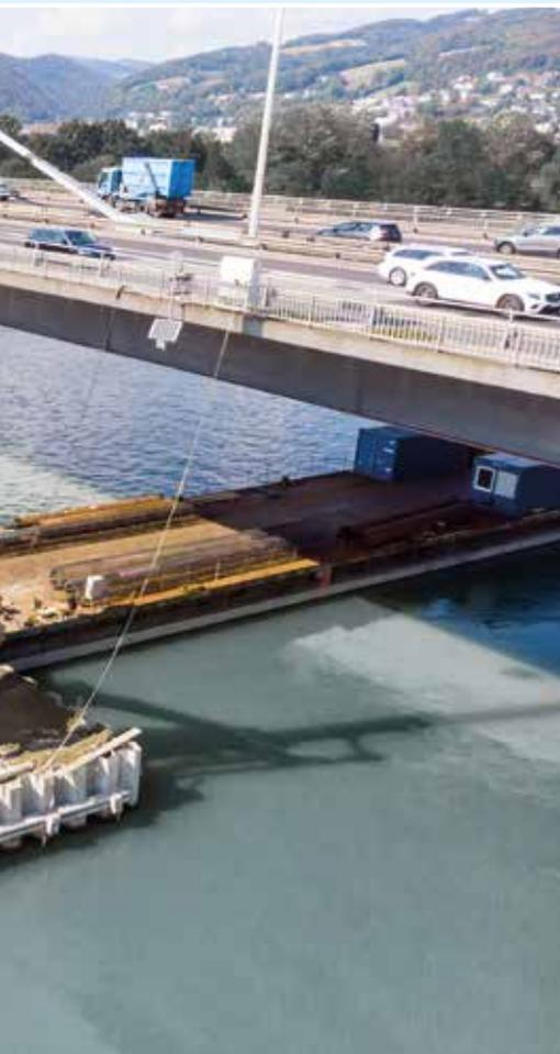
**Austria** For remediation and enhancement of the road safety of a highway bridge over the River Danube in Linz, around 10,000 m of piles were installed. For the deep foundations of a total of four pier sites for two bypass bridges, Bauer also drilled approx. 1,600 m piles inside sheet pile wall boxes, which were previously installed in the River Danube. **Left**
