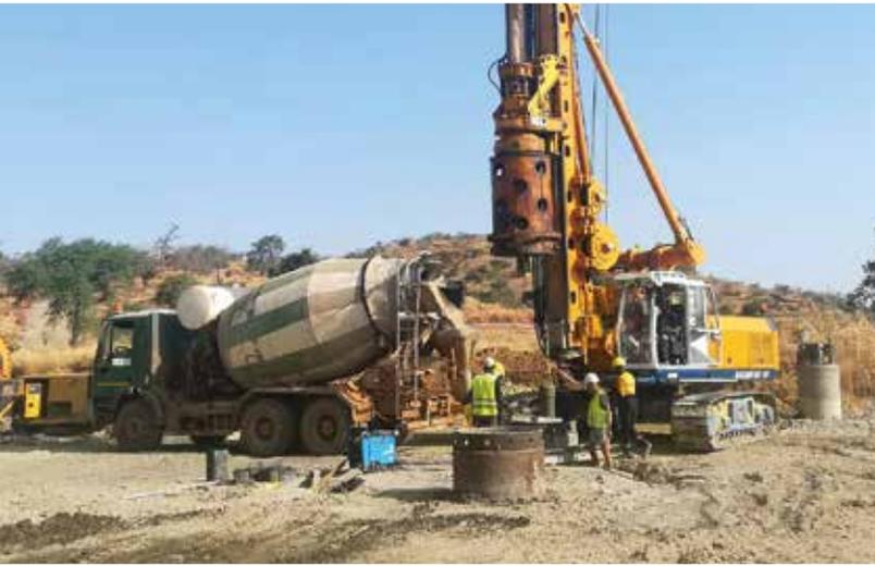
**Qatar** For the new Red Line of Doha's subway system, 333 tube-à-manchettes were drilled and installed for the purpose of filling in a total of roughly 4,000 m<sup>3</sup> injection material to stabilize the soil. **Bottom**
