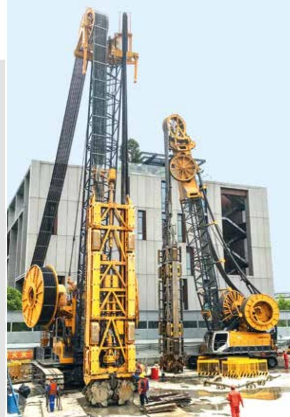
**China** In the Chinese metropolis Shanghai, our customer Shanghai Tunnel used a BC 40 cutter on an MC 96 duty-cycle crane, as well as a BC 50 cutter on an MC 128 duty-cycle crane. **Top**
