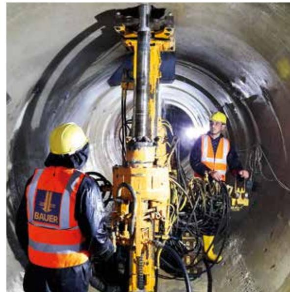
**Lebanon** Bauer already completed the works for the Jannah Dam, north-east of Beirut, in 2017. Roughly 20 drainage bores with a length of between 5 and 35 m were drilled retrospectively in the dam's drainage tunnel. **Top**
