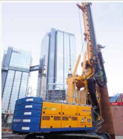
**Sweden** For the subway in Gothenburg, our customer Aarsleff is building a secant pile wall using a BG 36 H. **Top**
