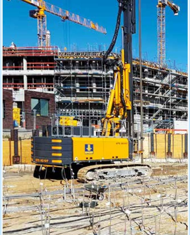
The underground car park for the major project at Quartier Heidestraße in **Berlin** is being built in a trough excavation pit, with walls being produced using the mixed-in-place method. Bauer is carrying out the horizontal sealing of the approx. 16,000 m<sup>2</sup> excavation pit in the form of a silicate gel base using an RG 19 T. **Top**
