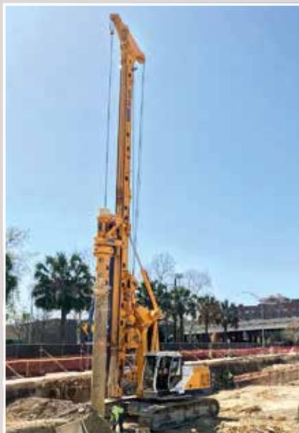
**Norway** Oslo-based YIT Norge AS used an RM 20 pile driver to install 72 piles measuring 914 mm in diameter to depths of up to 35 m for a new quay in Randaberg near Stavanger. The first piles were installed from the shore and subsequent piles were installed from a pontoon.
