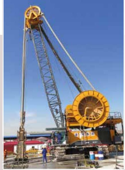
**China** Shanghai Foundation Engineering Group Co., Ltd. uses an MC 128 duty-cycle crane with a BC 40 cutter for an urban infrastructure expansion project in Shanghai.
