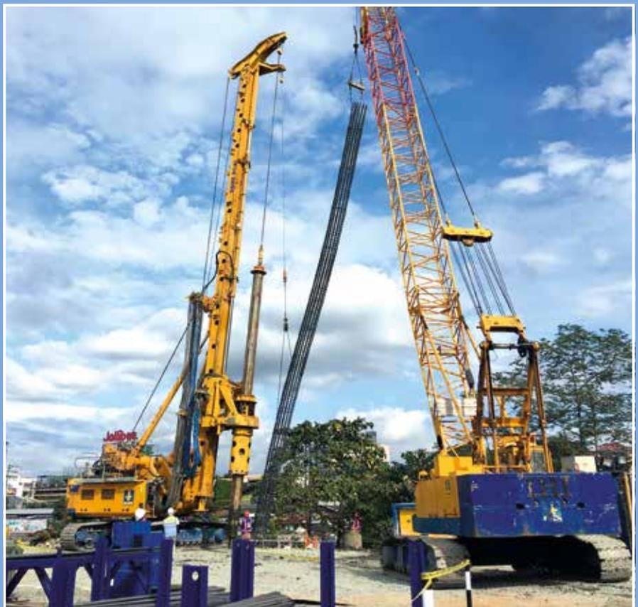
**Malaysia** Bauer installed bored piles with diameters of 1,350 to 3,500 mm in hard rock for an inner-city motorway bridge in Kuala Lumpur. The contract also included a test program consisting of a group of six test piles. **Above**
