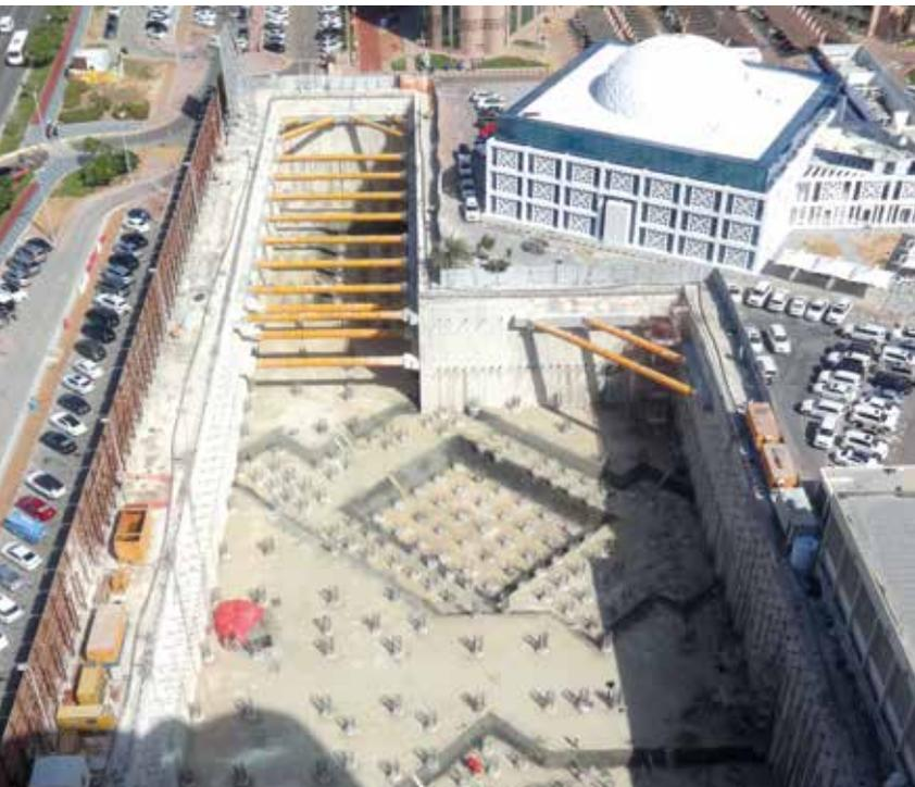
**Dubai** A gigantic shopping center is being built as part of the future Dubai II Big Box Retail Park. The excavation pit was constructed using secant and contiguous pile walls as well as soldier piles with wooden lagging over a length of 780 m. The project also included 1,754 foundation piles and 200,000 m<sup>3</sup> of excavation. **Right**
