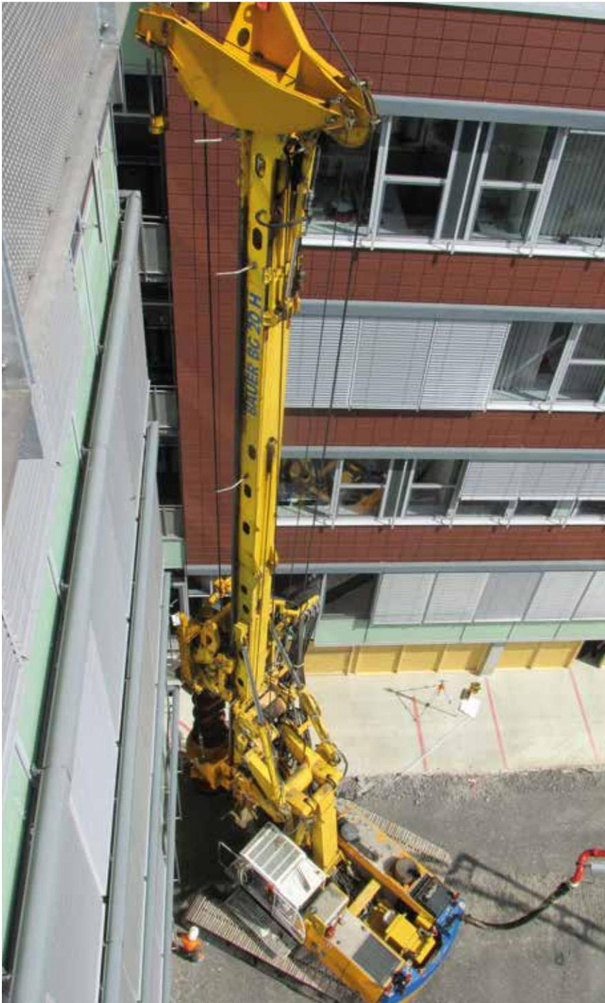
With space extremely restricted by neighboring buildings, a BG 20 H was used to install 64 CFA piles with a diameter of 750 mm up to 15 m deep in the ground for a new office building in **Weilimdorf**. **Above**
