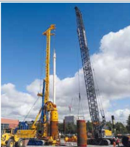
**Germany** A. Woehrl Spezialtiefbau GmbH used a BG 15 H with a BT 50 and Kelly drive for slope stabilization for a residential building in Freising.
