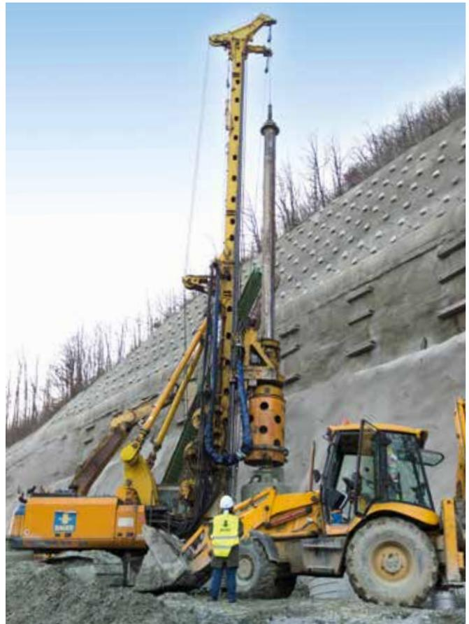
**Bulgaria** Between November 2017 and March 2018, Bauer's Bulgarian team used a BG 24 to construct 700 m of partially cased piles for a bridge section on the E75 highway near the Serbian town of Predejane. **Above**
