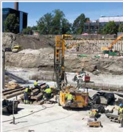
**China** Shenzhen Shenglong Construction Co. Ltd. uses a BCS 40 cutter to build Niuhu Station on Shenzhen Metro Line 4.
