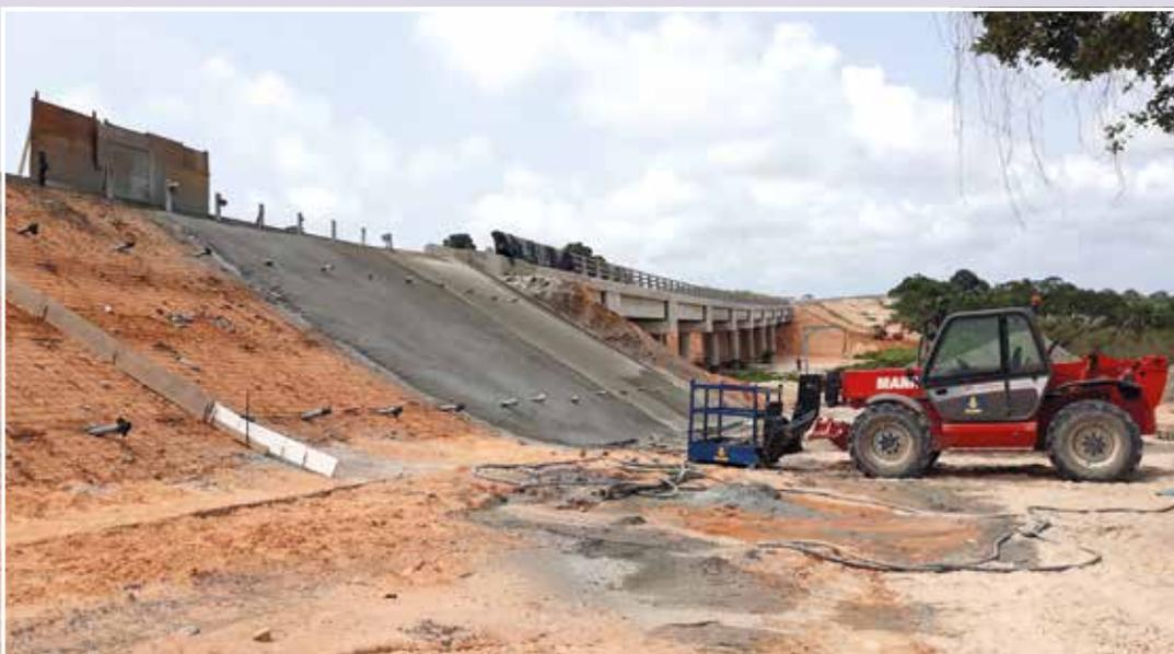
**Angola** Between December 2017 and March 2018, 4,000 m<sup>2</sup> of shotcrete and 500 m of soil nails were inserted to stabilize the slope along a road embankment. **Left**
