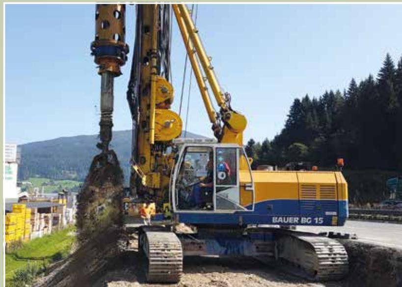
**Austria** On the A10 Tauern motorway south of Salzburg, noise barriers are being built on a foundation consisting of 9,900 m of bored piles. Two BG 20 H and BG 15 drilling rigs are being used. **Above**
