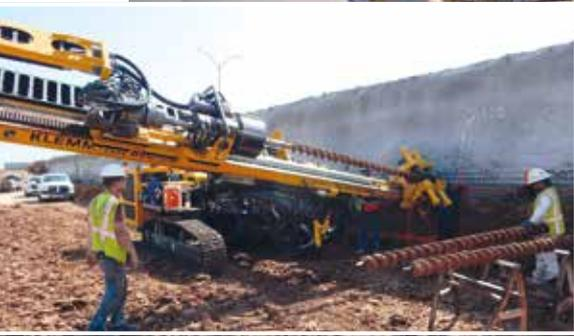
**USA** Our customer Malcolm Drilling used a CBC 25 cutter and a MAT BE 550 desander for slope stabilization below the Prado dam on the Santa Ana River in Corona, California for the construction of a concrete diaphragm wall.
