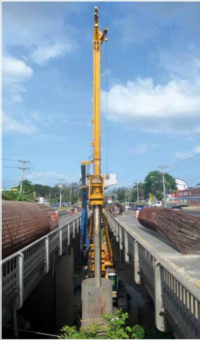
**Panama** From January 2016 to March 2018, a BG 28, BG 39 and BG 40 were used to install 783 bored piles up to 2,250 mm in diameter to depths of up to 43 m for the foundation of the continuous elevated metro line 2 in Panama City. **Left**
