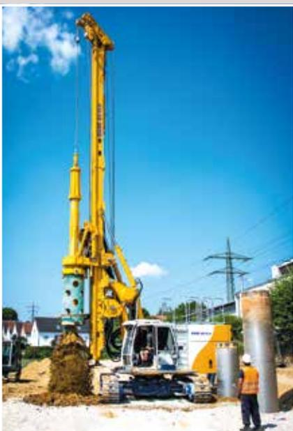
**Austria** Vienna-based Porr Bau GmbH uses a BG 45 in Kelly drilling mode to construct a bridge foundation that is 24 m deep and 1,500 mm in diameter for a town bypass in Oberau, Bavaria.
