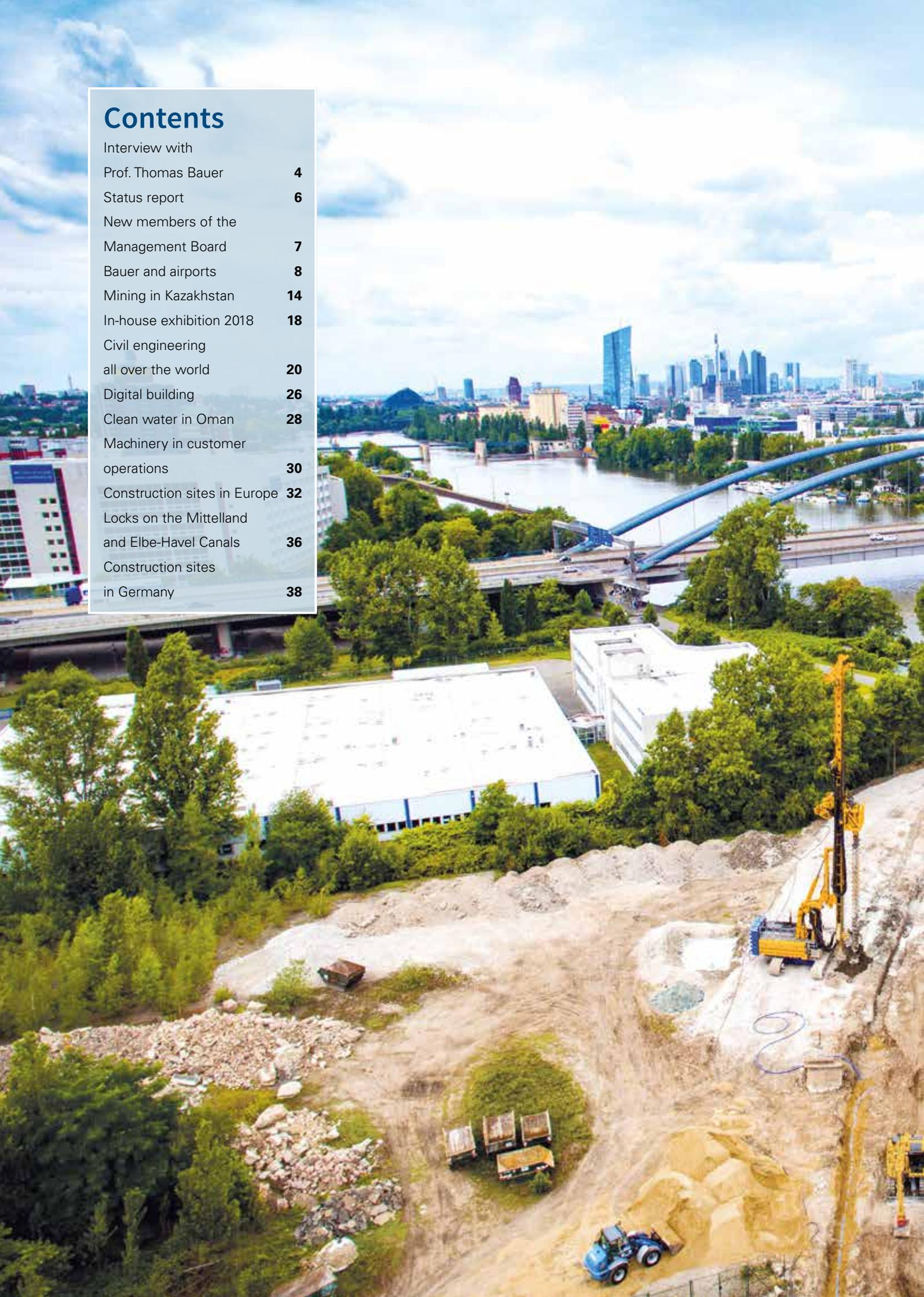
*A former tar factory in Offenbach is being remediated in several stages, including encapsulation with Mixed-in-Place walls and closure of gaps using the HPI method and sheet piles.*
