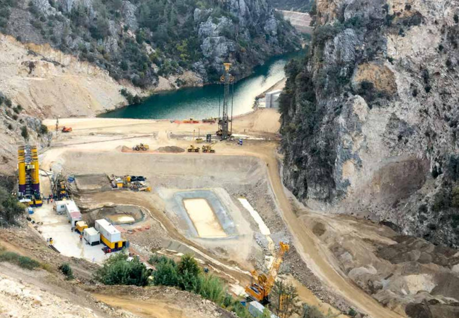
**Lebanon** Bauer was contracted to reinforce the Jannah dam. Cutter excavated diaphragm wall panels were installed to depths of up to 50 m to create a bentonite concrete cut-off wall along a 123 m stretch of the dam. **Above**
