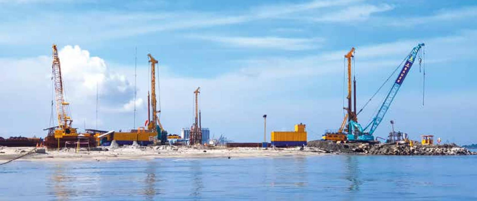
**Indonesia** Bauer built a secant pile wall and anchor piles for a port being planned on an artificial island two kilometers off the east Indonesian city of Makassar Sulawesi. **Above**
