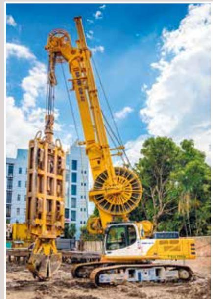
**Sri Lanka** San Piling Pvt. Ltd. uses a GB 40 grab to construct diaphragm walls for a real estate project in the capital city of Colombo.
