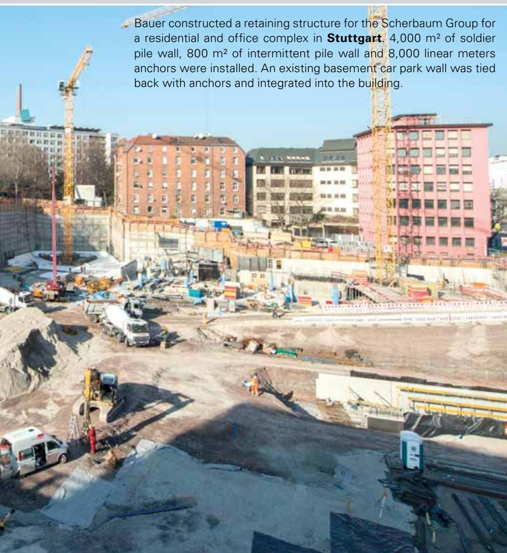
Bauer constructed a retaining structure for the Scherbaum Group for a residential and office complex in **Stuttgart**. 4,000 m<sup>2</sup> of soldier pile wall, 800 m<sup>2</sup> of intermittent pile wall and 8,000 linear meters anchors were installed. An existing basement car park wall was tied back with anchors and integrated into the building.
