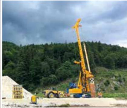
**Estonia** Our customer Baltpile OÜ used three BG 30, BG 36 V and BG 40 V specialist foundation engineering rigs and a KR 806 anchor drilling rig to construct the excavation pit for a multifunctional building complex in the Tallinn yacht harbor.
