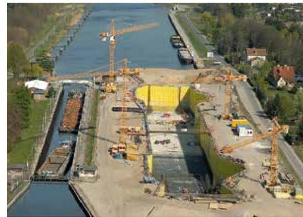
*The sheet piles of the cut-off wall for the new Wusterwitz lock were covered with a material called Pecafil.*
