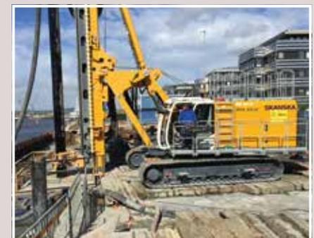
**USA** Schnabel Foundation Company in Texas uses a BG 20 H to install piles measuring 610 mm in diameter up to 9 m deep into the ground for an office building in San Antonio.
