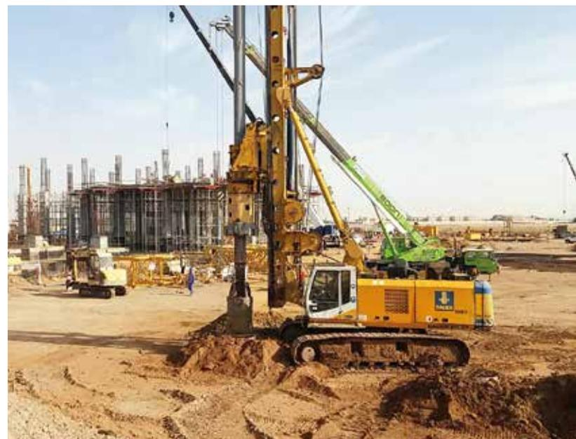
**Saudi Arabia** In Dhahban, near Jeddah, Bauer completed three large contracts for the Security Forces Medical Center between February 2017 and June 2018. Two BG 40 and six BG 28 were used to perform eight pile tests and construct 2,000 wall piles and 4,600 foundation piles. **Above**
