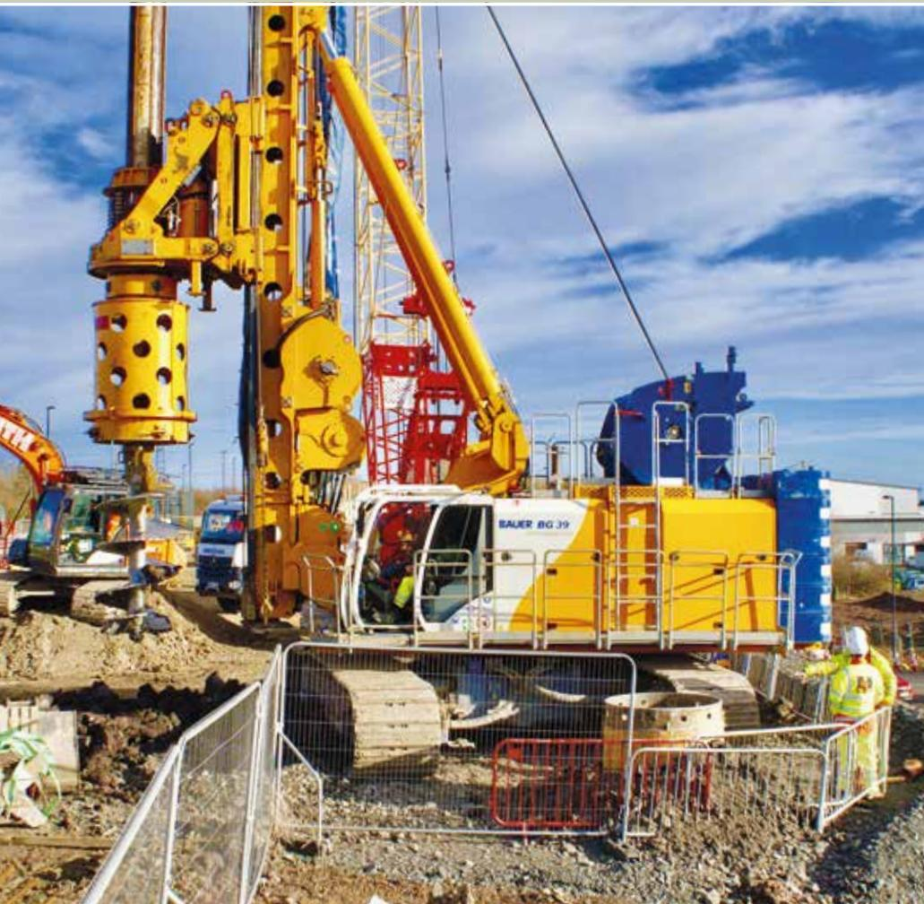
**England** The junction of the A19/A1058 motorways at Newcastle is being converted into a new triple-decker interchange junction. The excavation pit for the underpass of the A19 and the foundations for the abutment of three bridges consists of 600 bored piles that are 1,500 mm in diameter and 31 m long. The work was carried out in two phases where there was with flows of heavy traffic ongoing. **Above**
