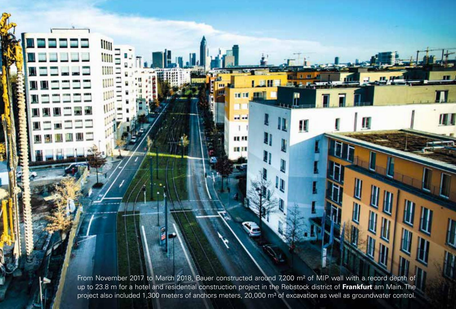
From November 2017 to March 2018, Bauer constructed around 7,200 m<sup>2</sup> of MIP wall with a record depth of up to 23.8 m for a hotel and residential construction project in the Rebstock district of **Frankfurt** am Main. The project also included 1,300 meters of anchors meters, 20,000 m<sup>3</sup> of excavation as well as groundwater control.
