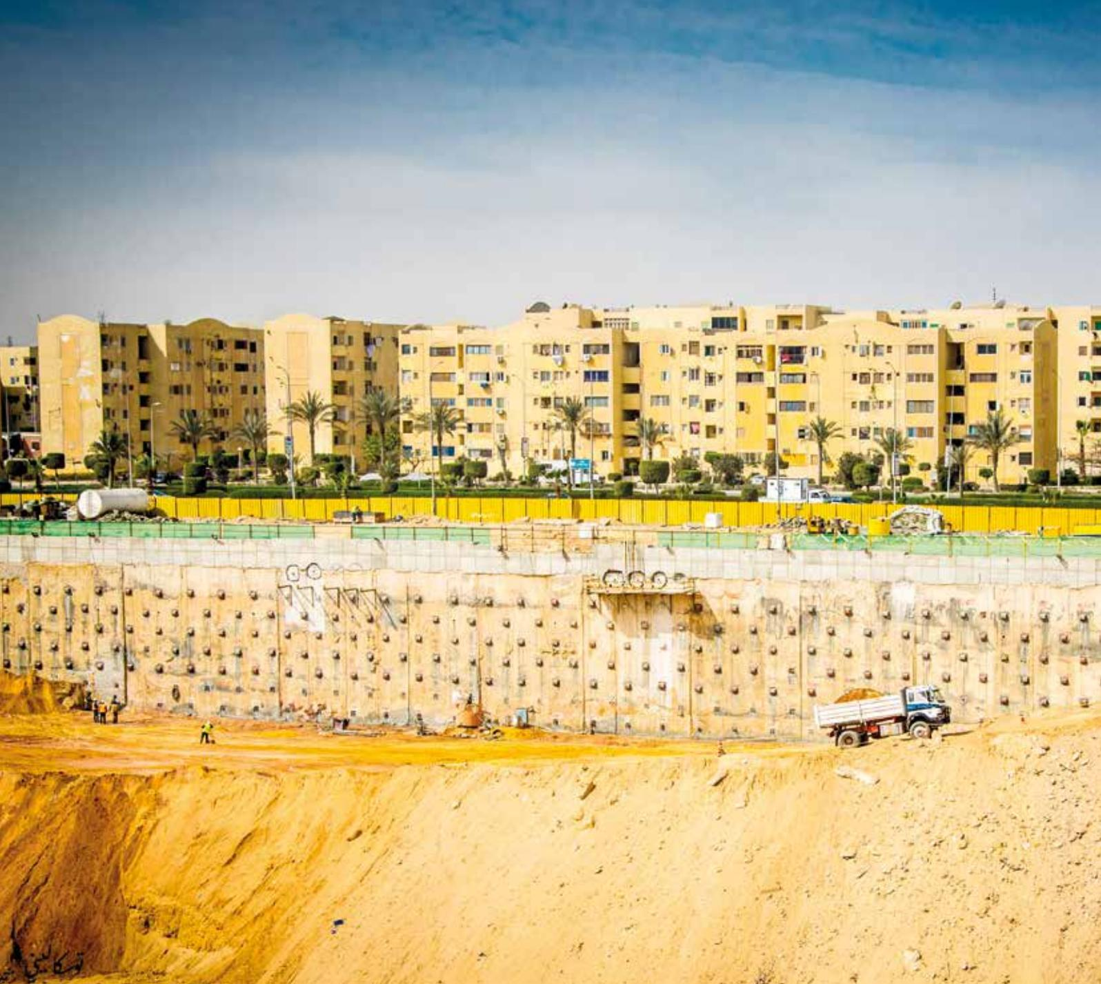
**Egypt** From September 2017 to March 2018, a BC 30 cutter and a Klemm 806 anchor drilling rig were used to construct a diaphragm wall tied back with anchors 27 meters deep and 800 mm in diameter for a 17-meter-deep excavation pit at the Cairo Cancer Hospital. **Above**
