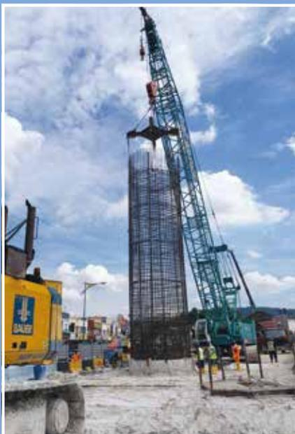
**Philippines** Sixty-five 2.8 m diameter bored piles were installed on land and seventy-four 3.4 m diameter offshore piles were installed in the San Juan Riverbed for the extension of the Metro Manila Skyway. The maximum depth of the piles is 44 m. **Below**
