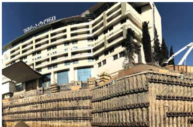
**Georgia** Bauer was subcontracted to install three layers of anchoring for existing pile wall for the foundation of the basement car park and casino at the Sheraton Hotel in Tbilisi. **Above**
