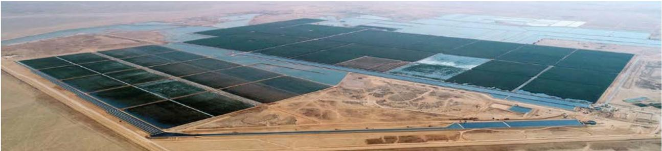
The plant-based purification facility in Oman not only cleans 175,000 m<sup>3</sup> contaminated water daily, but the reduction in CO<sub>2</sub> emissions also meant that emission certificates for 114,000 t of CO<sub>2</sub> could be sold in 2019.
