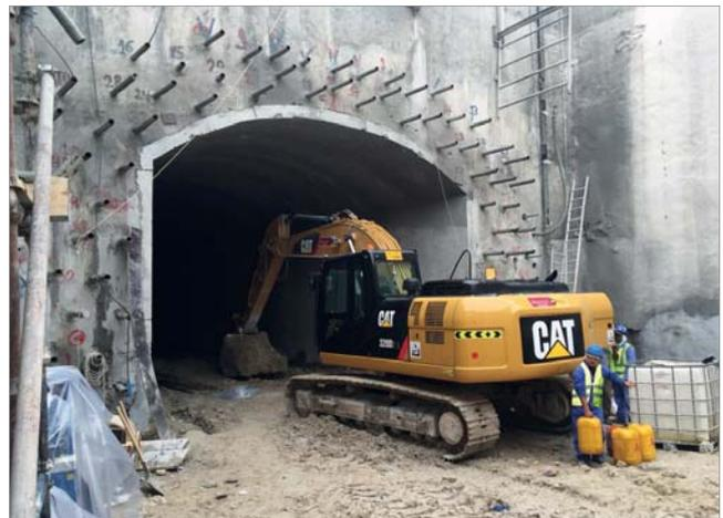
Pedestrian underpass in Abu Dhabi, UAE: Tunnel with TaM pipes
