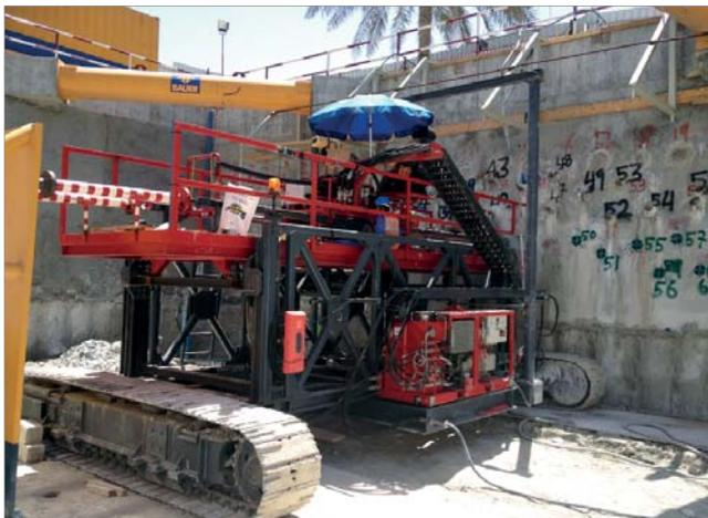
Pedestrian underpass in Abu Dhabi, UAE: HDD guided drilling
