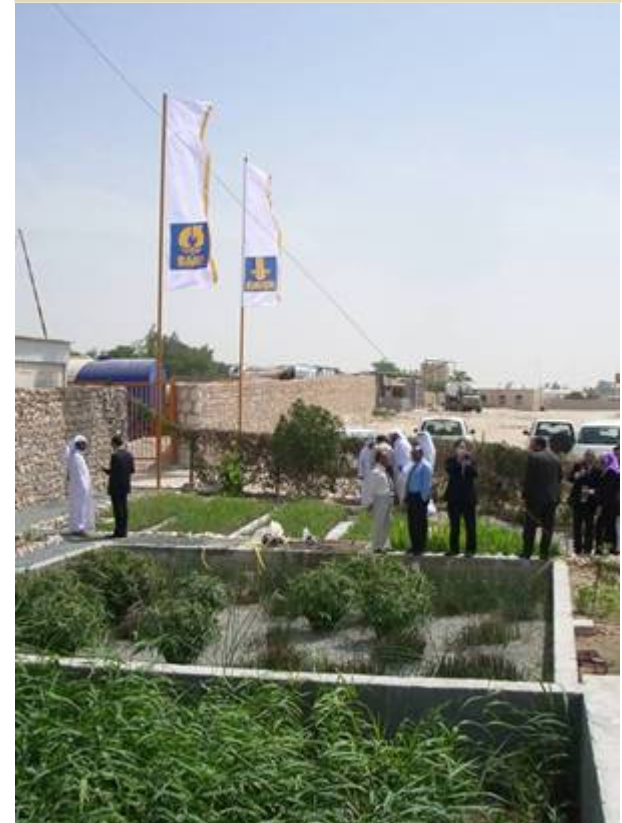
Plant-based sewage treatment works, Abu Dhabi
