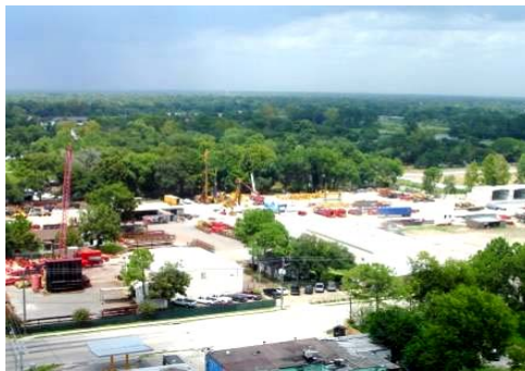
Pileco, Houston, Texas, USA
