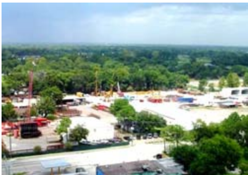
Pileco, Houston, Texas, USA
