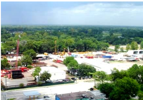
Pileco, Houston, Texas, USA
