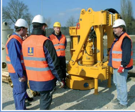
Instruction in machinery proficiency – the rotary drive is the main component for drilling.
