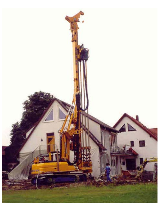
Cut-off wall with BG, Oberhausen, Germany
