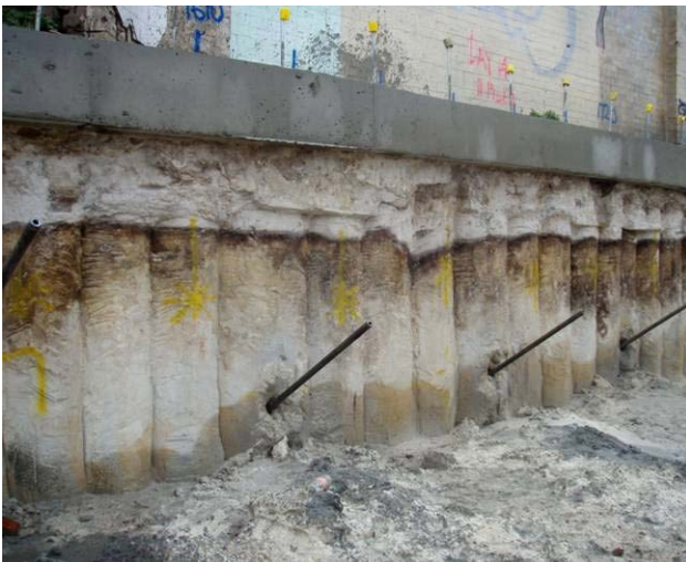
Excavated SMW retaining wall, Sydney, Australia
